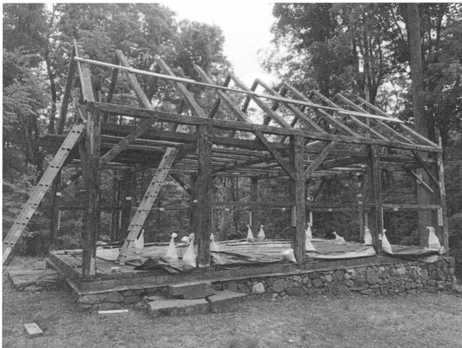
Roof Rafters Completed
