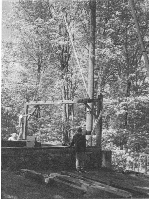
First Vent Raised
